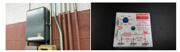
Conduit from the breaker box may already exist and will lead to an enclosure box near the dishwasher for the hood motor control. If this is not the case, it will need to be provided. From the ADS Hood Fan Kit, install this relay next to the fan motor contactor. Wire according to wire diagram supplied in kit.
