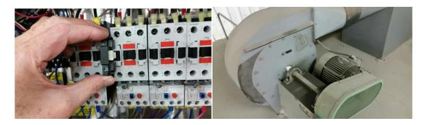
Next, inside the dishmachine's control box, insert the slave points (291-3028) on the conveyor motor contactor for conveyor machines and the wash contactor for the HT-25. Wire according to wire diagram supplied in kit.
